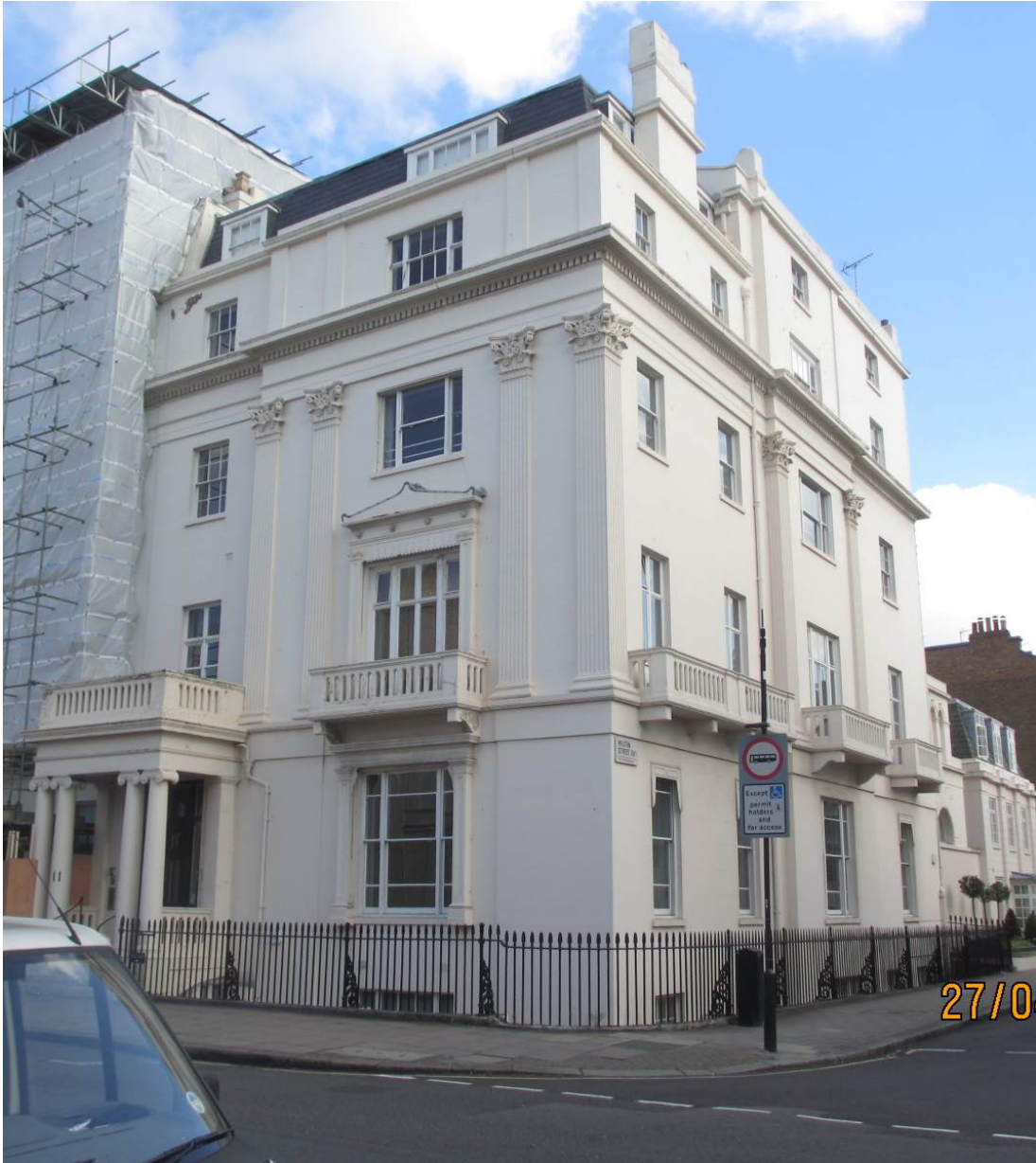
Photo 1: Upper Belgrave Street (front) and Wilton Street (side) elevations
