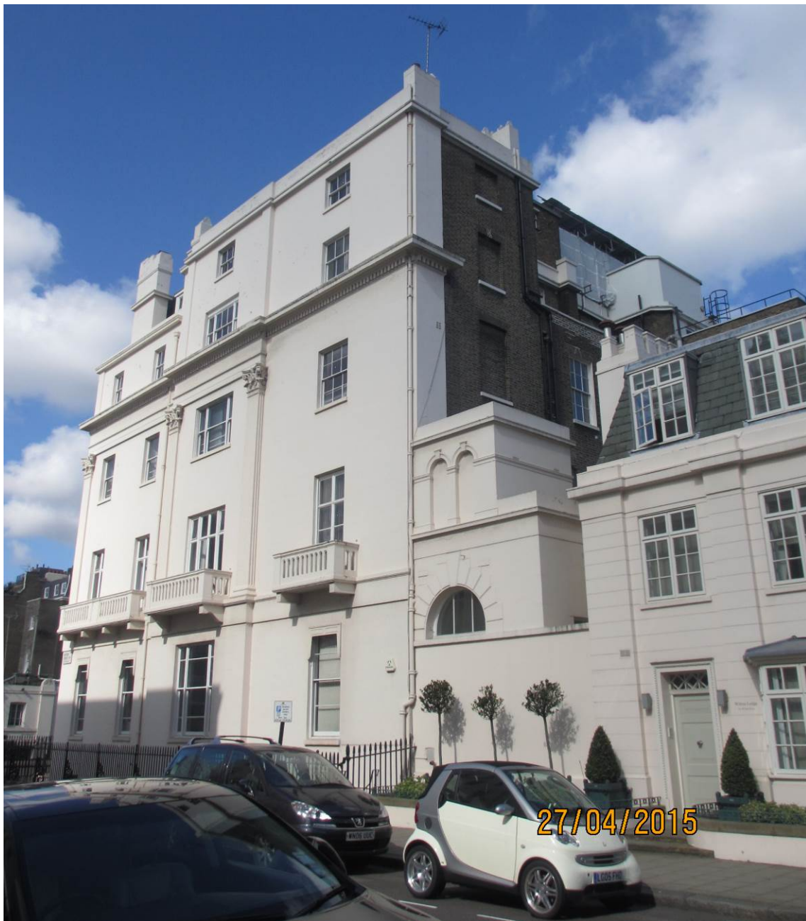
Photo 2: Wilton Street (side) and Wilton Mews (rear) elevations, showing main rear wing, currently faced in brick with a stucco return, with the lower closet wing adjoining to the right.
