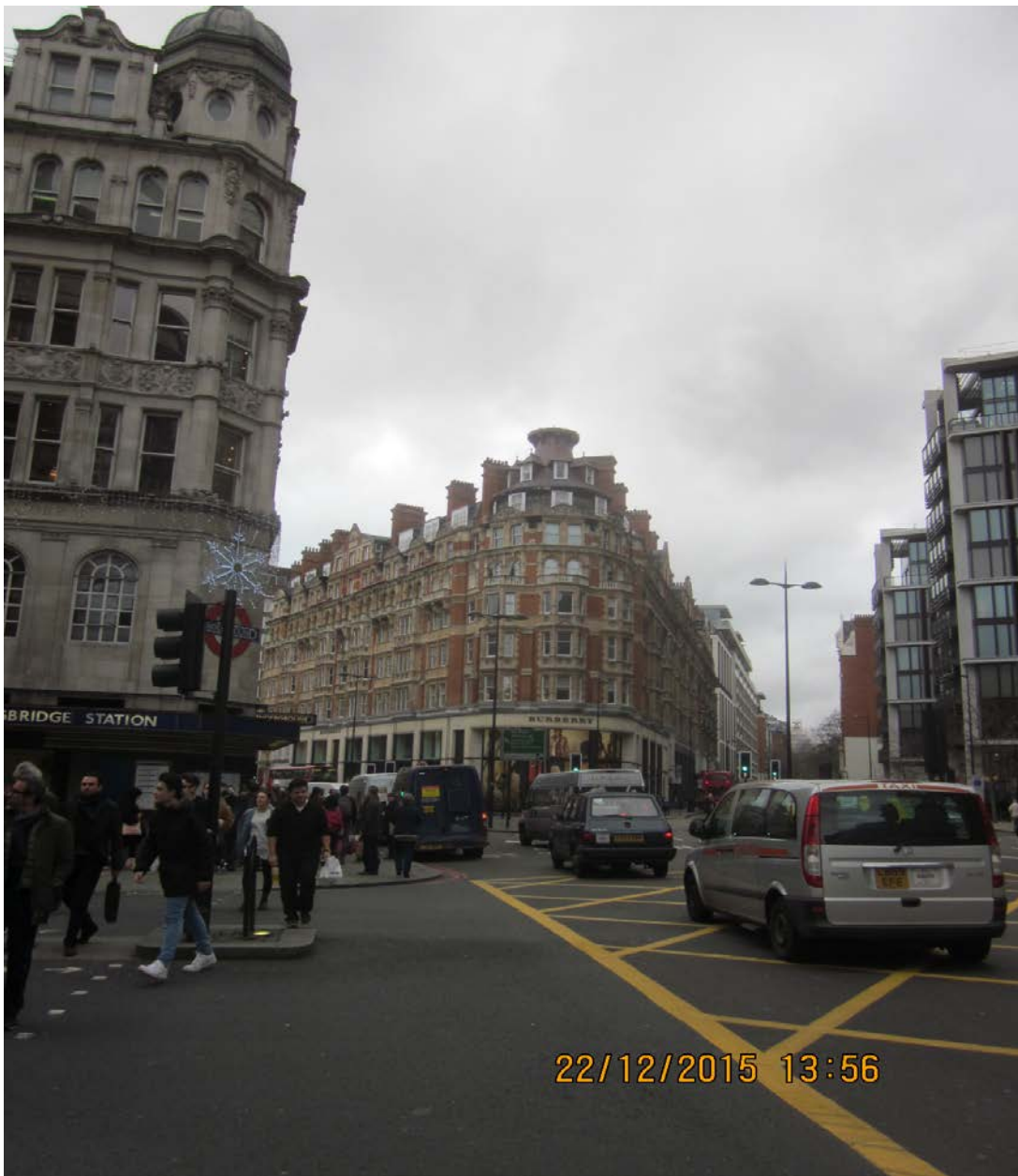
Long View from the east
